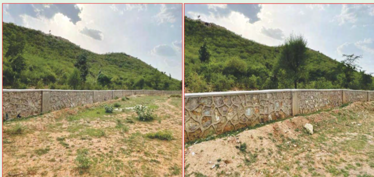
Ecorestoration wall 4 feet at Jhiri forest block in Alwar
