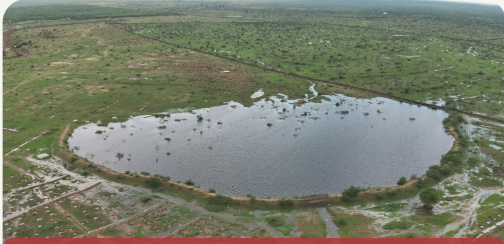
MPT and soil & moisture conservation works in the afforestation plot at Shankarpura Choki, Kota—planned and implemented by the field team using skills gained from basic and advanced SMC training
